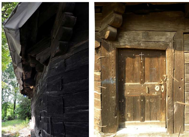
Fig. 1 – a. Dovetail joints and decoration of consoles; b. The door from north side of narthex.
