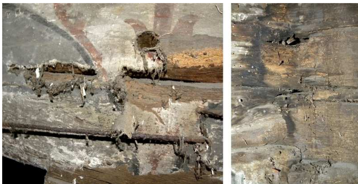
Fig. 6 – a. degradation of interstitial canvas; b. Degradation of beams – inside the church
